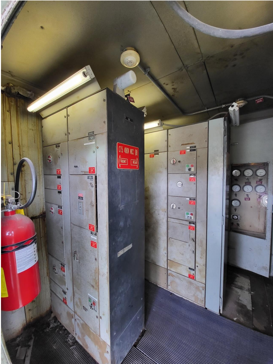
Current CT5 cab – northern half (showing LV MCCs)
