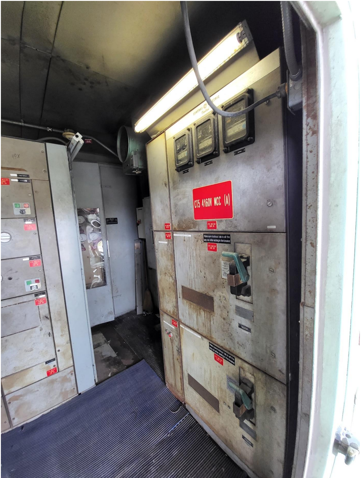
Current CT5 cab – southern half (showing MV MCC and heater)
